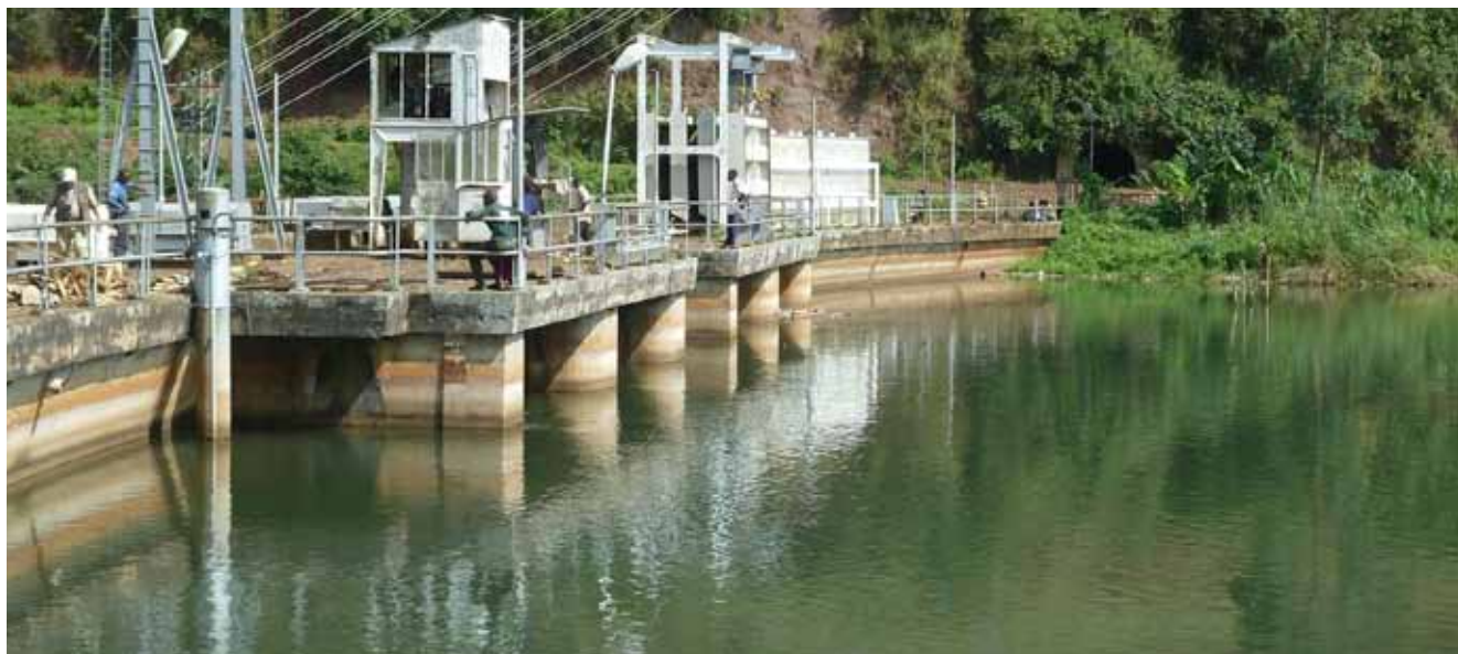
hydroelectric power plant project along River Ruzizi
