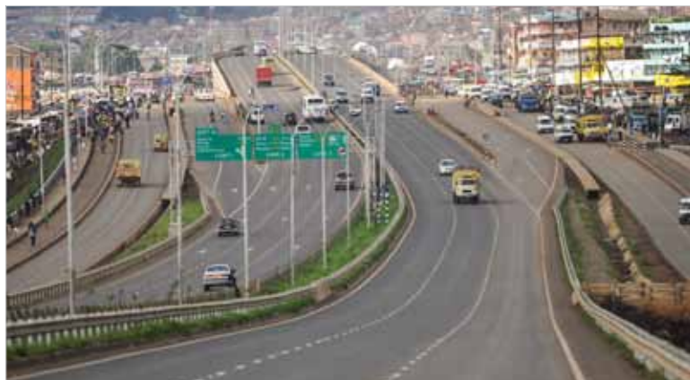
A section of the Thika Super-highway
